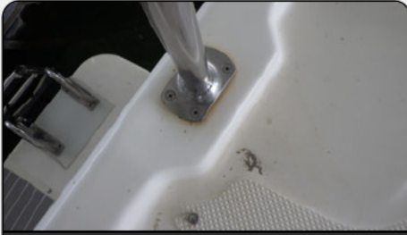
Photo 12: corrosion on the stanchion mounting.
