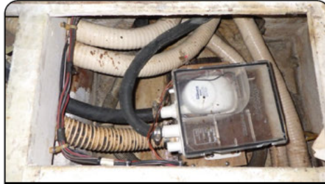
Photo 40: View of fwd shower sump
