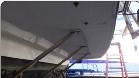
Photo 6: Rusted fasteners need replacing with marine grade stainless steel
